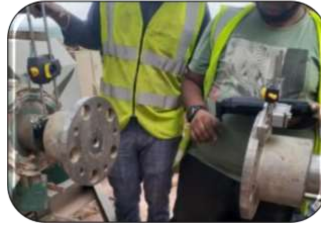
Laser alignment at site
